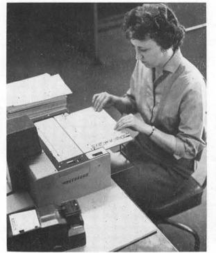
PERSONNEL RECORDS, vital documents, and Technical Library manuals are photographed on 16mm film by this Recordak camera operated by Bonnie Smith. Special feature is the complete film unit which attaches to the camera. An average of 2300 shots is taken on 16mm reels each day.
